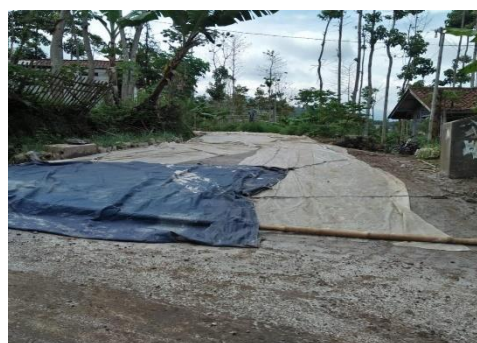
Figure 1. Improvement of the Mekarlaksana Village cast road
